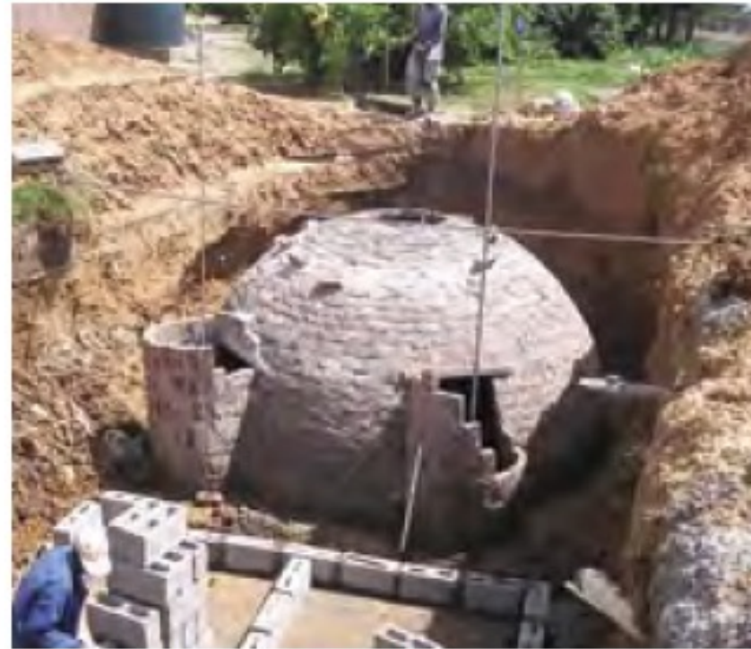
Picture 9: Fixed-dome digester under construction in Lesotho (photo: Sandec).
