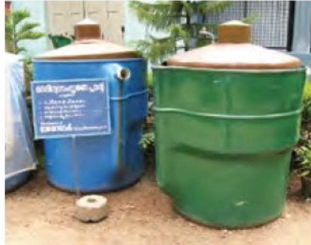
Picture 11: Above ground floating-drum digester for households in India, made of fibreglass reinforced plastic (photo: Sandec).
