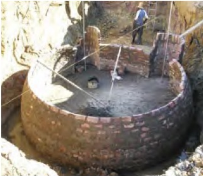
Picture 9: Fixed-dome digester under construction in Lesotho (photo: Sandec).
