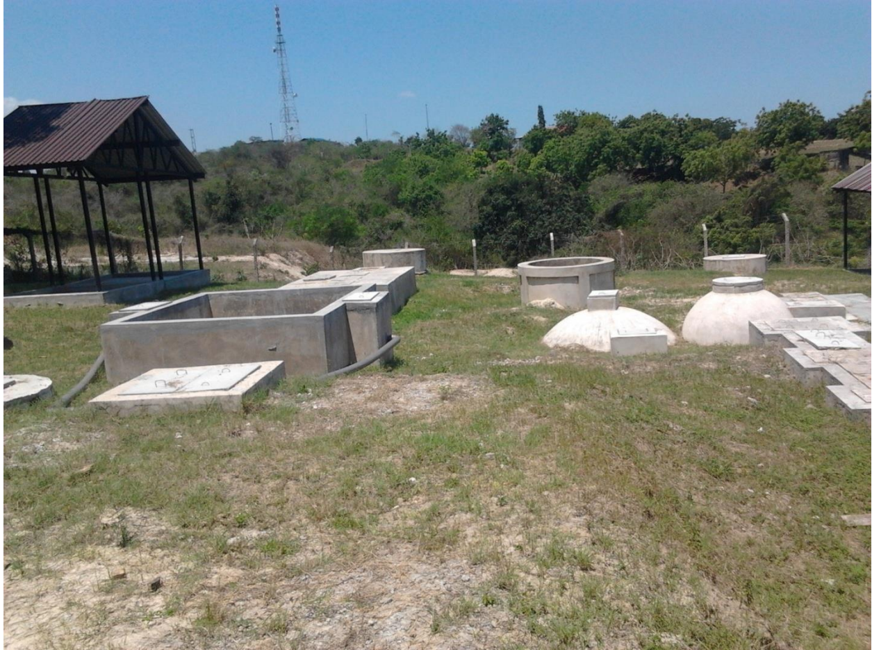
Figure 7.3: Another view of the IWM&RR constructed on ARU campus in Dar es Salaam. In the middle ground towards the left edge of the picture can be seen an upflow anaerobic sludge blanket (UASB) reactor. The two pipes that are visible on the right and left sides of the UASB reactor are for delivery of influent from the chamber which is right in front of the UASB reactor. The chamber receives effluents from a hydrolysis reactor (partially visible in the picture) which processes effluents from a solid waste size reduction and homogenisation unit (not visible in the picture).
