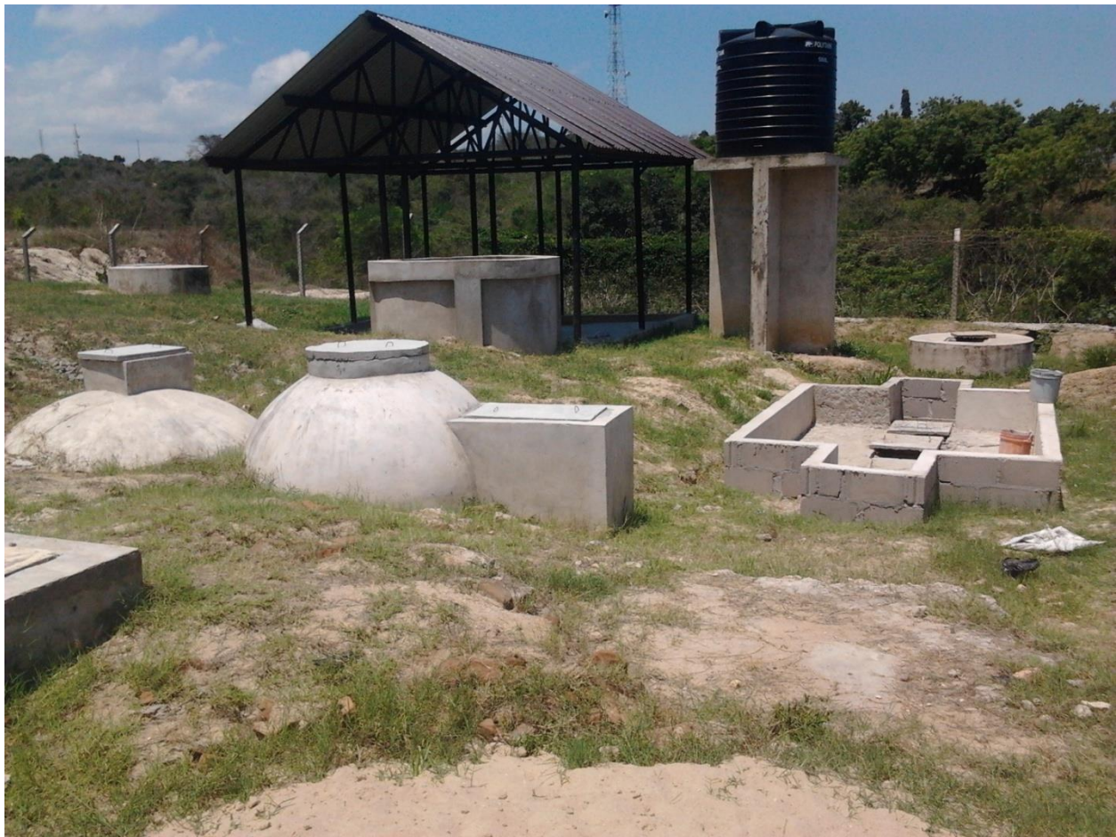
Figure 7.1: A view of the IWM&RR constructed on ARU campus in Dar es Salaam. In the middle right side of the picture is an anaerobic baffled reactor (ABR) while a biogas digester is to the left of the ABR. An underground tank for treated waste is right behind the ABR while an elevated tank for treated wastewater is to the left of the underground tank. A unit for biogas storage is located right behind the biogas digester. A sludge and slurry processing unit is located behind the biogas storage unit to the left of the treated water elevated storage tank. In the background the fencing poles which are visible demarcate and physically separate the irrigation plots from the rest of the IWM&RR system units which can be seen in the middle of the picture.
