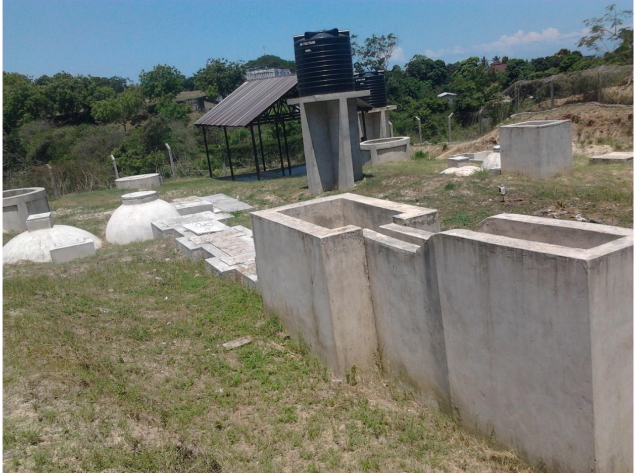
Figure 7.2: Another view of the IWM&RR constructed on ARU campus in Dar es Salaam. In the foreground towards the right hand side corner of the picture can be seen a faecal sludge receiving unit which is connected to a flow equalisation unit towards the middle of the picture. A covered channel for delivering the faecal sludge extends between the sludge flow equalisation unit and the biogas digester towards the middle of the picture slightly towards the left edge of the picture. An elevated water storage tank is to the right of the biogas digester behind which can be seen the sludge and slurry processing unit. Slightly behind and to the right of the elevated water storage tank can be seen a biogas storage unit. Further to the right of the elevated water storage tank towards the right top corner of the picture can be seen a solid waste pre-digestion processing unit (for size reduction and homogenisation)
