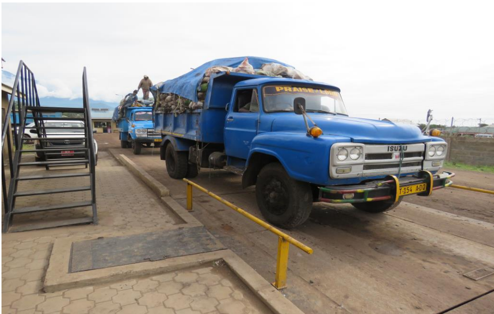
Muriet Landfill Weight Bridge – Arusha City Council
