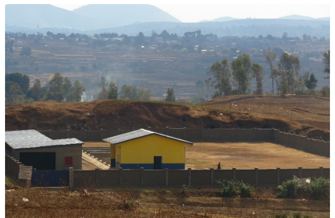
View of the platform for composting waste and plastic recycling (NE side of the landfill)
