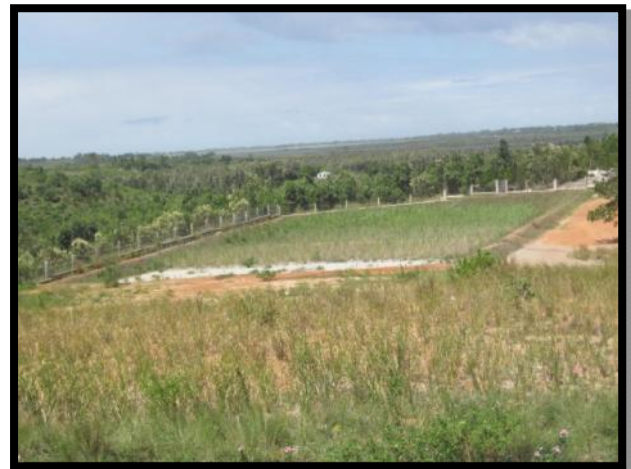
ANKAREFO: LEACHATE TREATMENT BASIN
